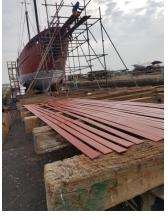
Above, the ship with her new bowsprit under construction and the completed work, below, much stronger than before with larger chain and cable stays. The flat bar seen here is for use repairing the rusted bulwarks on the main deck.
